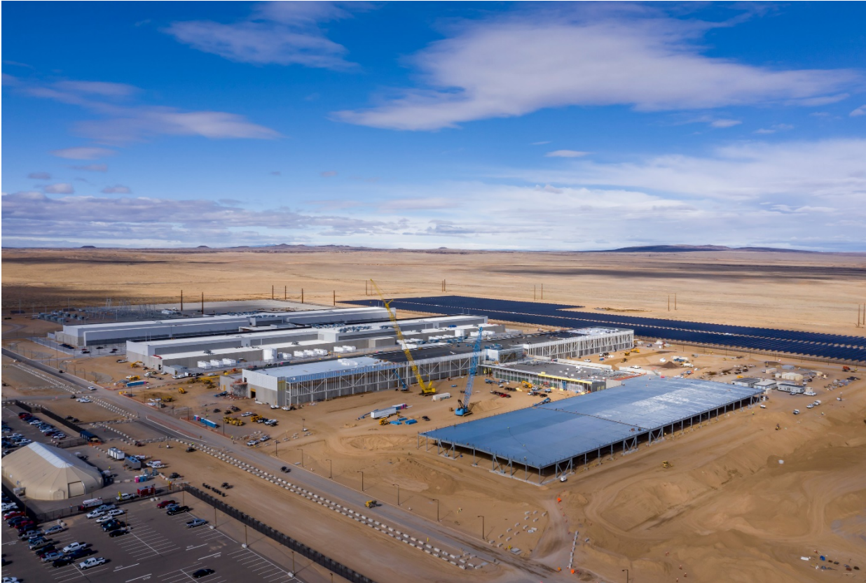
Figure 2 Facebook Data Center in New Mexico
