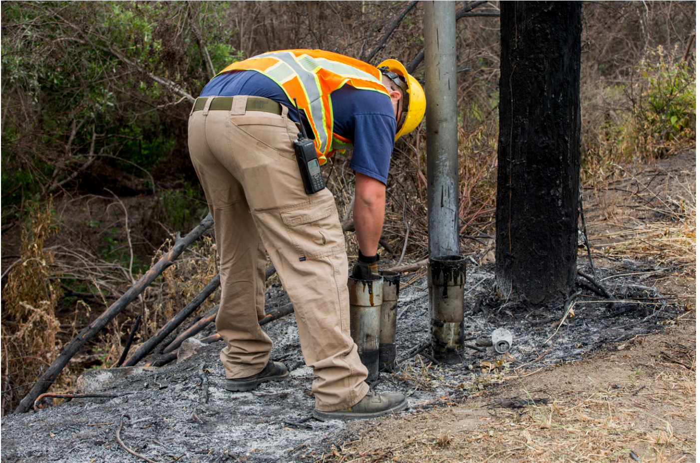
Figure 6. Base Telecom employee assesses fiber optic cable damage after wildfire at Camp Pendleton, CA (Image: Sft. Luis Vega, Wikimedia Commons )
