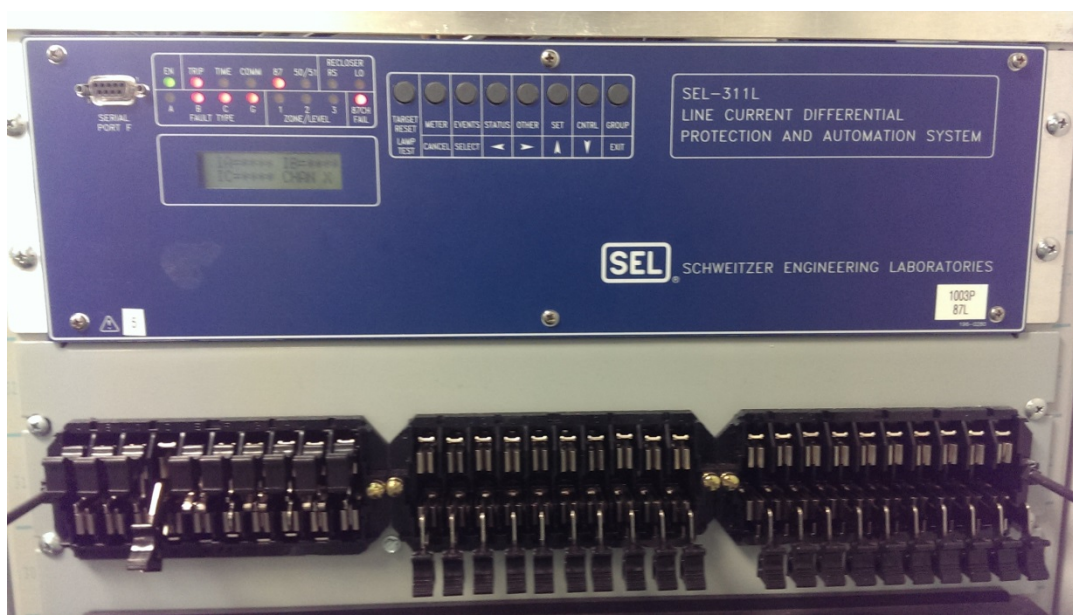
Figure 10 - Current Differential Relay
